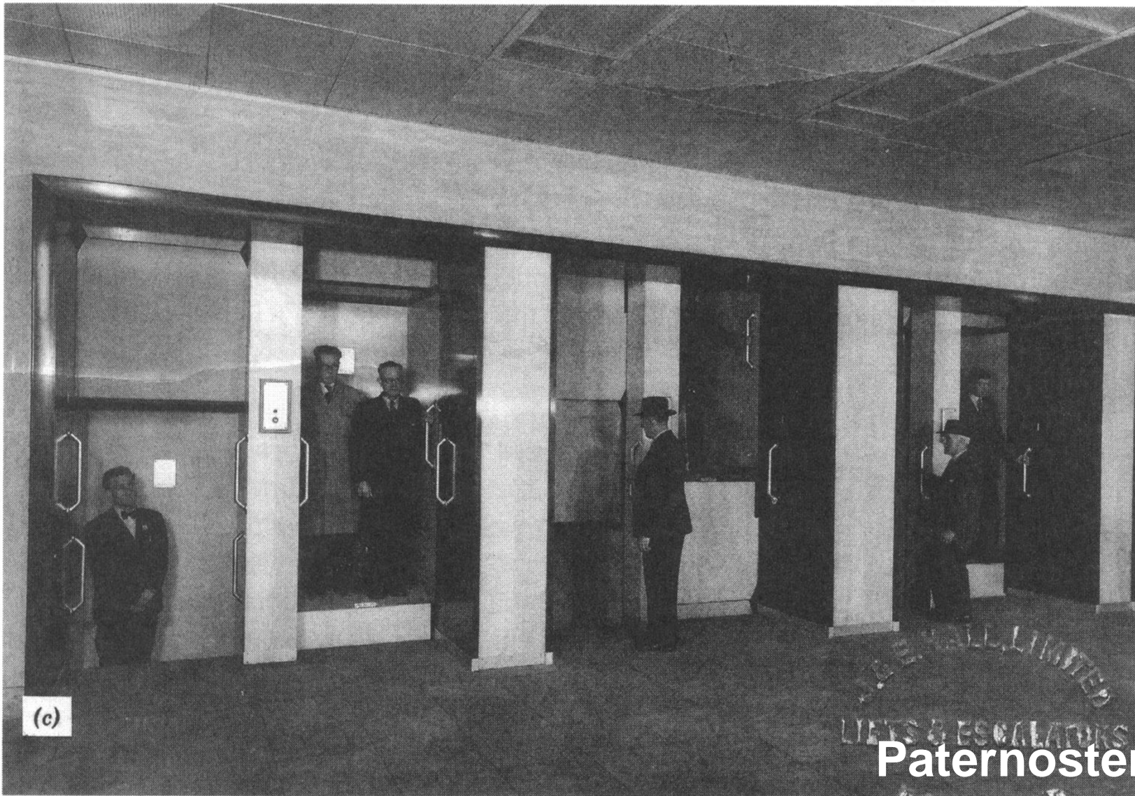
Figure 5.1. (Continued) (c) Actual installation.
