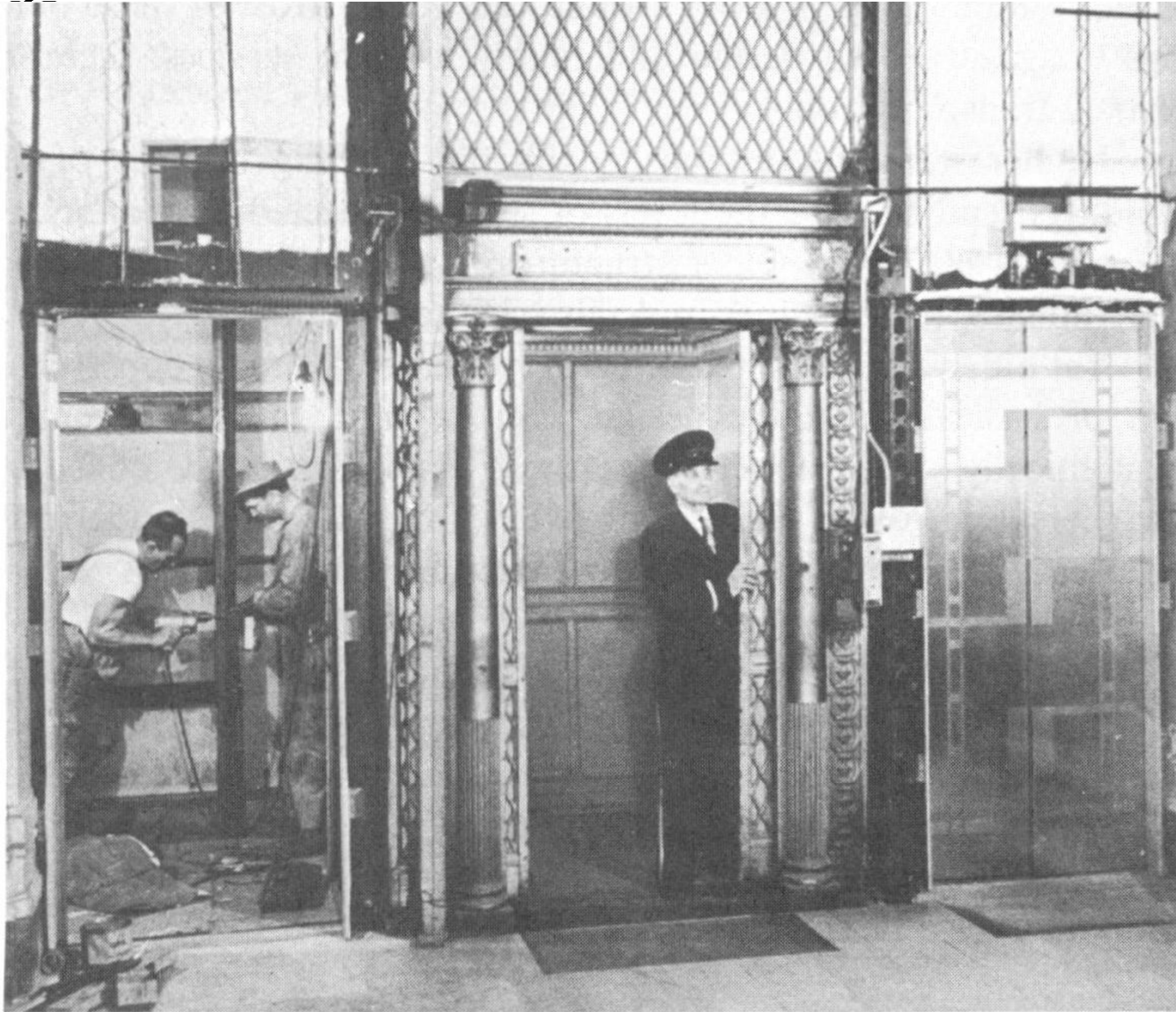
Fig. 12.1. Elevators being modernized while one car (center) continues in operation.
