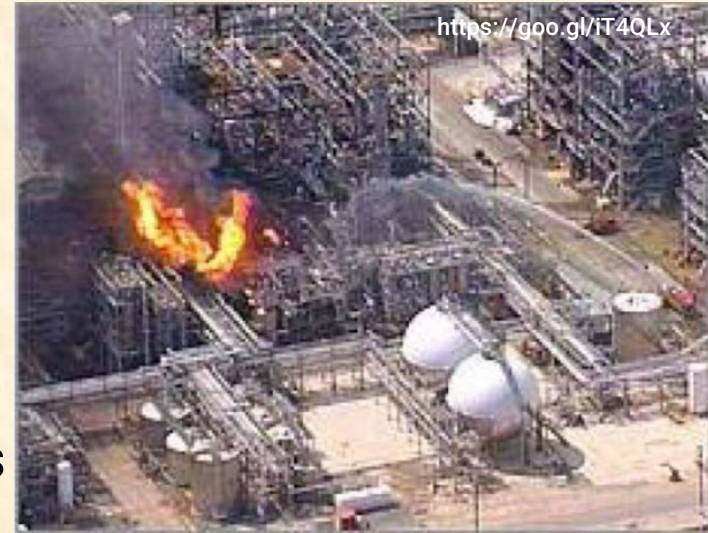
Figure 1. Accident Caused by SIF Failure
