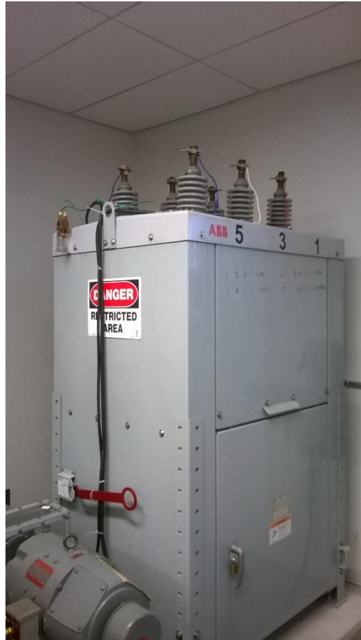
Utility Breaker 15kV ABB Vacuum Circuit Breaker
