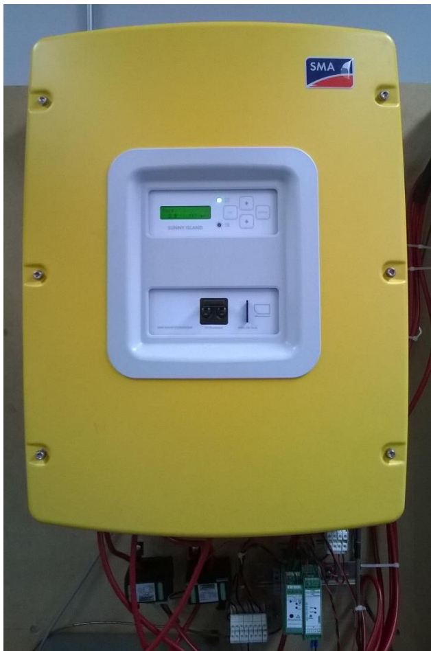
4.5 kW Bidirectional Converter/ Battery Charger SMA Sunny Island
