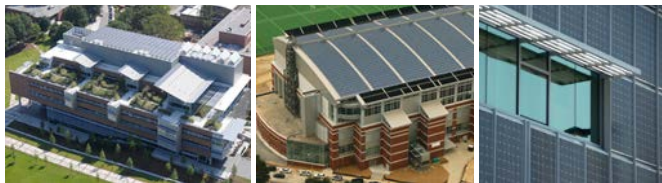
Fig. 6. PV Systems in the Smart Energy Campus Test Bed
