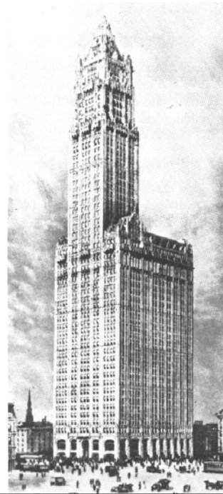
The 51-story Woolworth Building still has the Otis gearless traction machinery installed in 1912.
