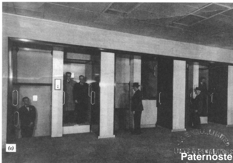
Figure 5.1. (Continued) (c) Actual installation.
