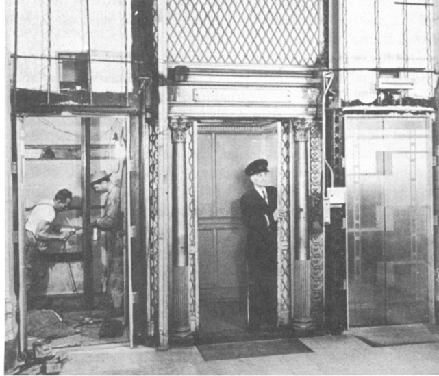
Fig. 12.1. Elevators being modernized while one car (center) continues in operation. [Strakosch98]
