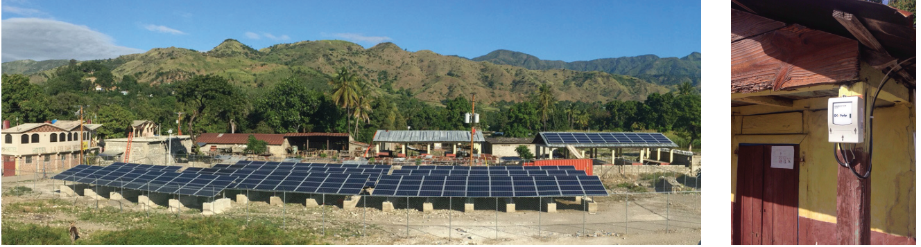
Figure 2: Solar PV array with battery and diesel generation (left) and Sparkmeter hardware (right)
