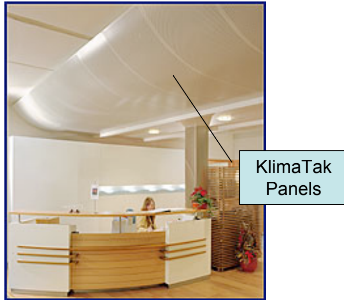
Figure 2.5: This picture shows a larger KlimaTak acoustical panel setup. These allow more space for infrastructure above the ceiling but otherwise are similar to the panels shown in Figure 2.3.
