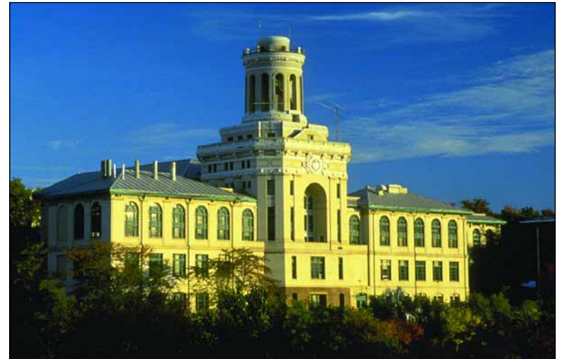
Carnegie Mellon's Nanofabrication Facility occupies space in the University's Hamerschlag Hall.
